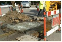
Image 14: The detected leak within 1m of model prediction (Source: DMU, 2015)
