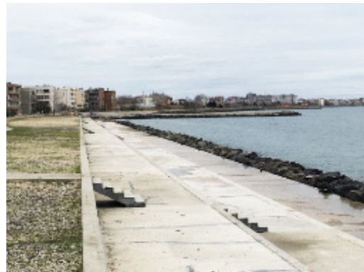
Coastal embankment to prevent flooding of a residential area. The height of the embankment can be increased in future if the flood hazard increases (Bulgaria)
